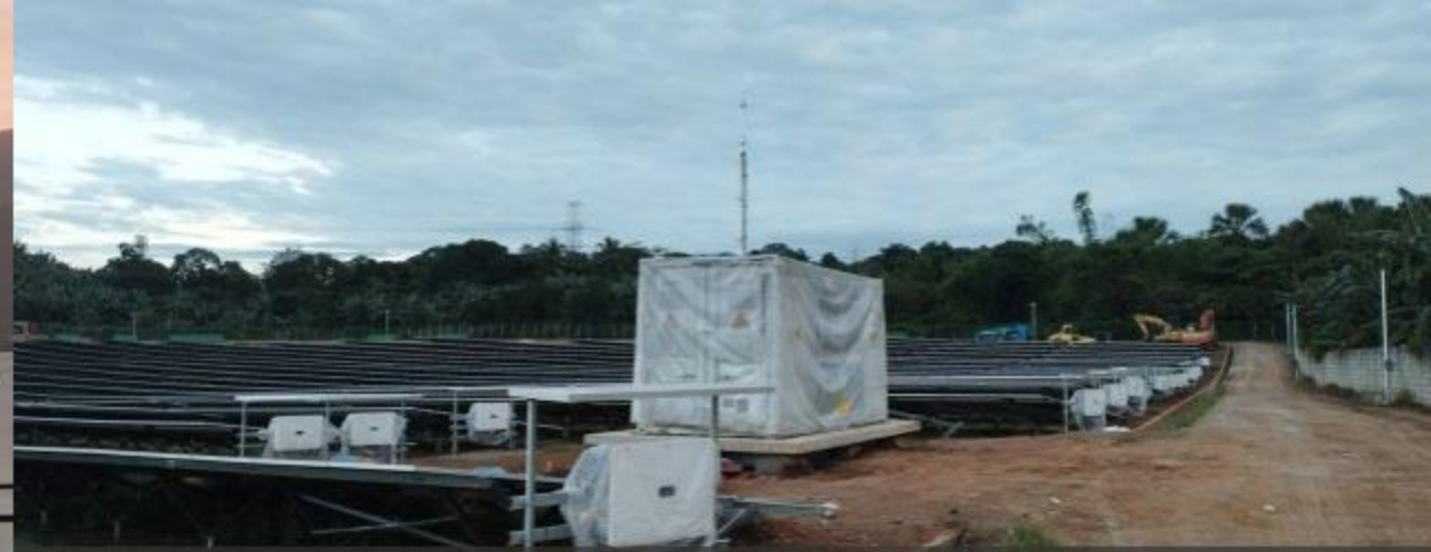
PAVI Bataan 20 MW Project Undergoing construction Implements a skid solution
