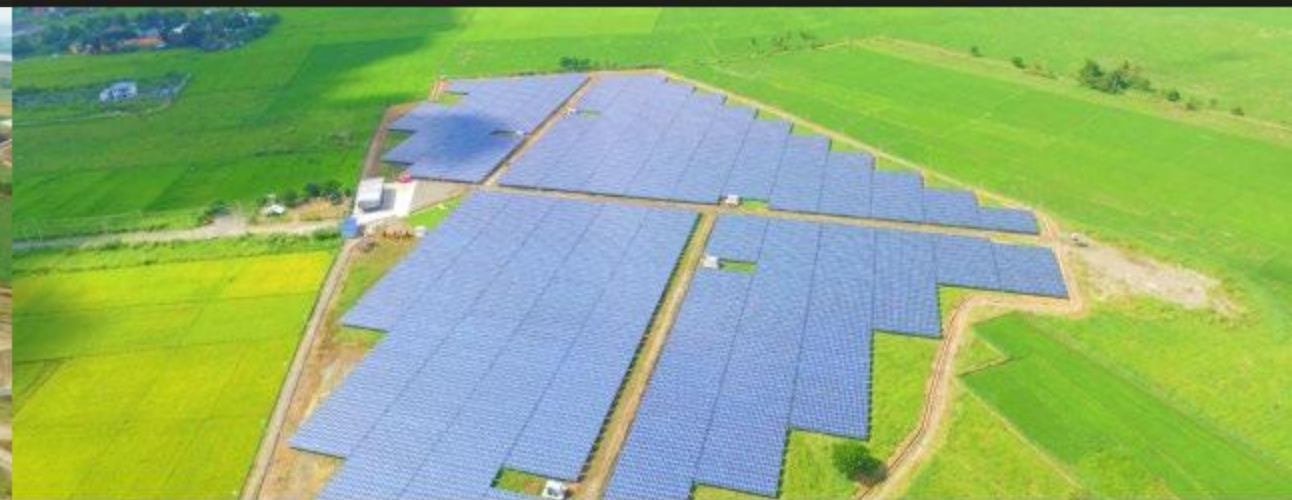
Cabanatuan 10 MW Project Located in Nueva Ecija 0.2% failure rate after 5 years
